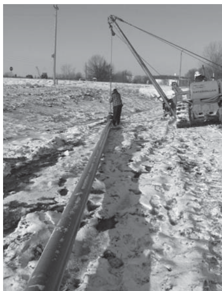
Construction crews work on a natural gas pipeline project near Carrollton.
